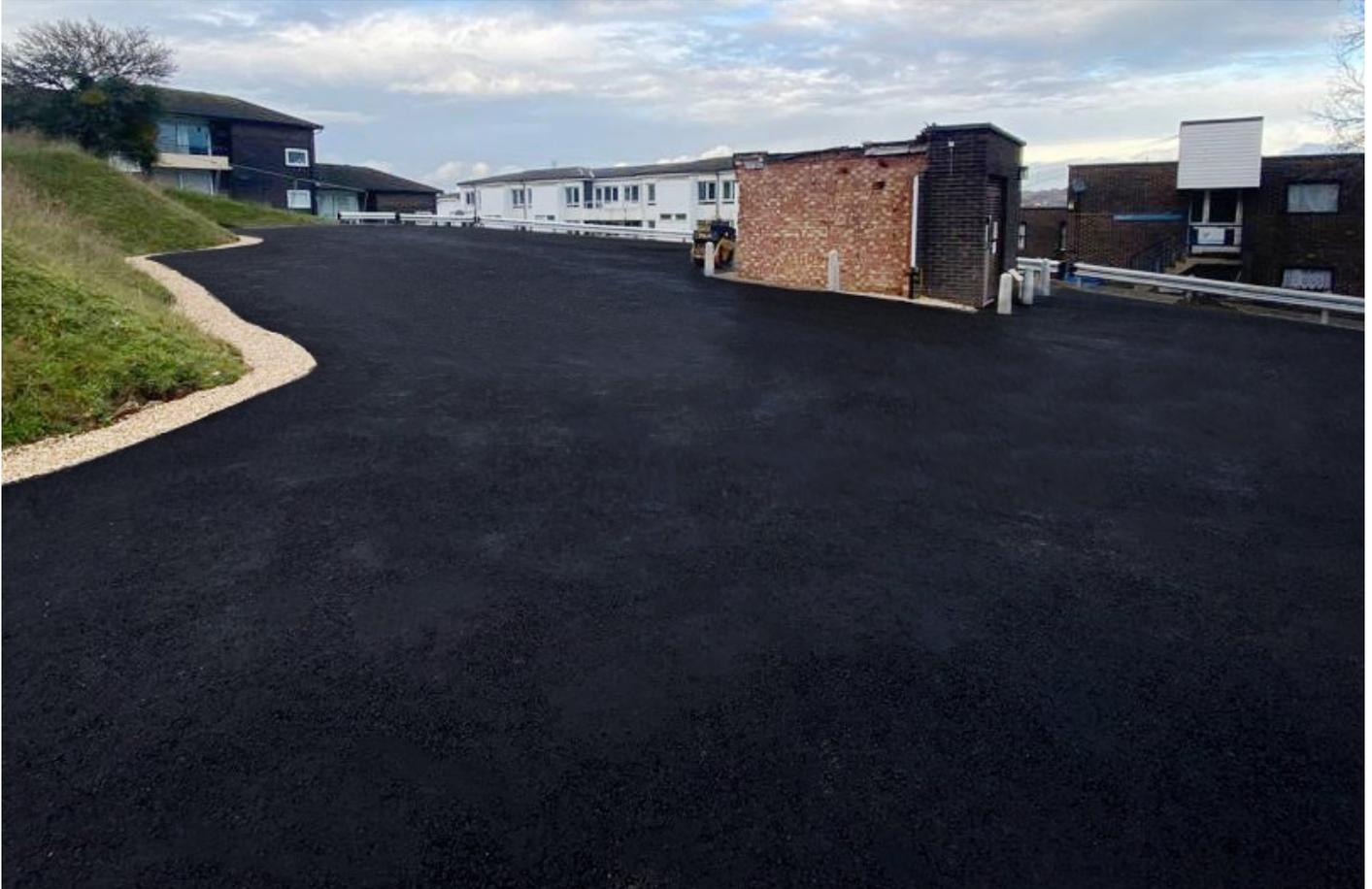
The £50,000 project included levelling the rough ground and removing vegetation before applying a substrate of type 1 aggregate. Tarmac surfacing was laid and marked with parking bay divisions, kerbs and edging established and areas of light-coloured gravel were used to enhance the aesthetic landscaping of the car park. Concrete safety bollards were also installed around an existing utilities hut to complete the well-planned car park design.
